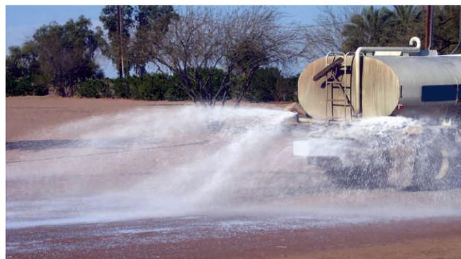
Dust control on road surface is done using Calcium / Magnesium Chloride or blended brines or frequent water spray. However, these treatments do not give any bonding to soil particles and get washed away during wet spell.
